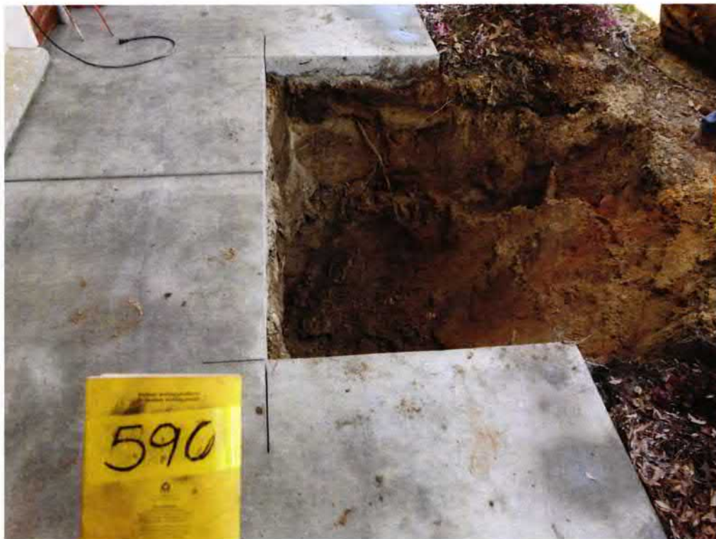
Picture 2: UST 590Aster excavation.
